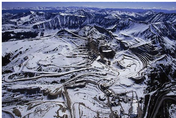
Climax molybdenum mine
