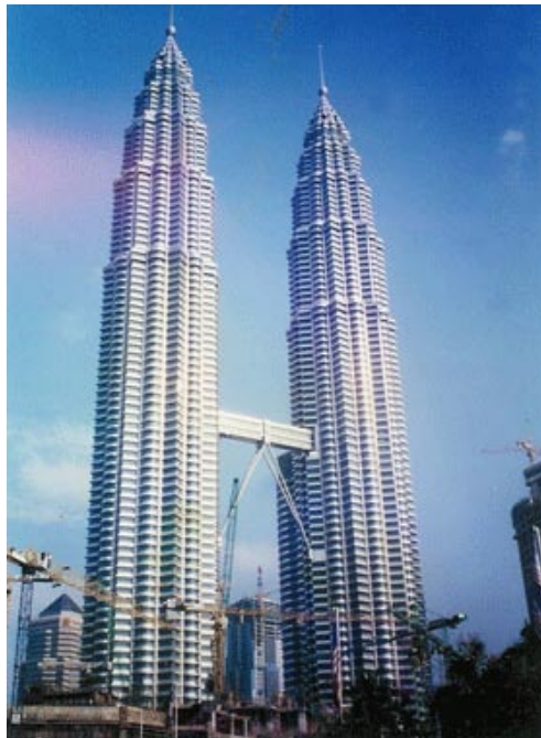
Malaysia's Petronas Towers, the world's tallest buildings, use a popular form of stainless steel, with a three percent molybdenum content.
